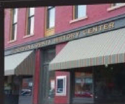
Jefferson County History Center
